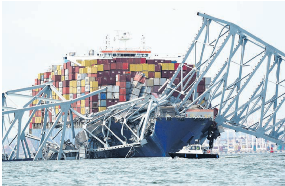
A cargo ship is stuck under the part of the structure of the Francis Scott Key Bridge after the ship hit the bridge Tuesday March 26, 2024, in Baltimore, Md.
